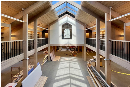
Second floor looking towards the front desk.
